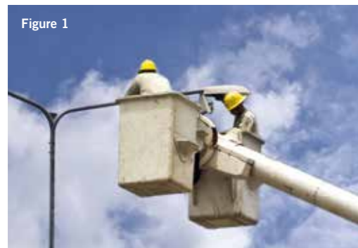
Figure 1 - Typical modern method to reach a lamppost.
